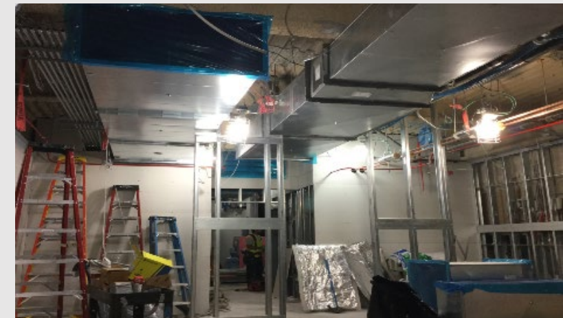
Installation – Overhead Duct & Utilities
