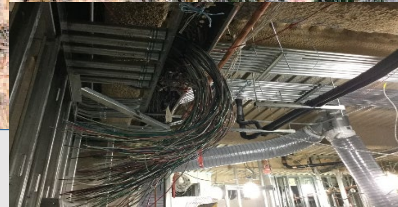
Relocation – Electrical to new Panels
