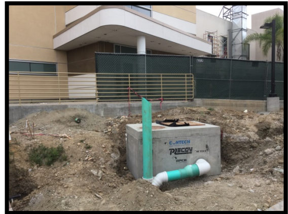
North Site Storm Water Vault Install
