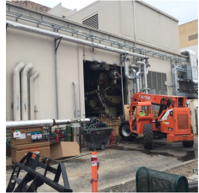
Demolition of Equipment in Existing Plant
