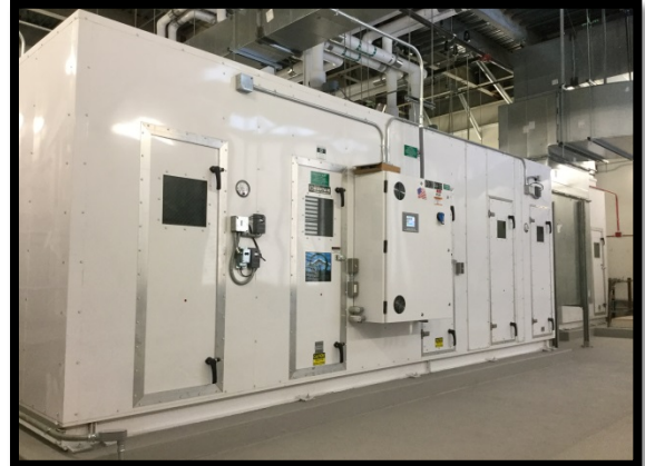
Level A AHU #22 Kitchen Tie In
