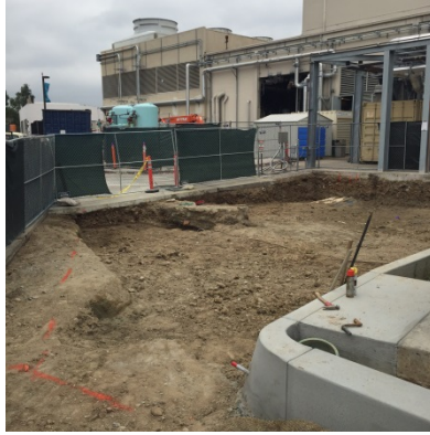
Excavation for new O2 Farm
