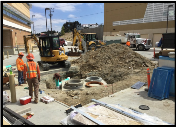
South Site Storm Water Vault Install
