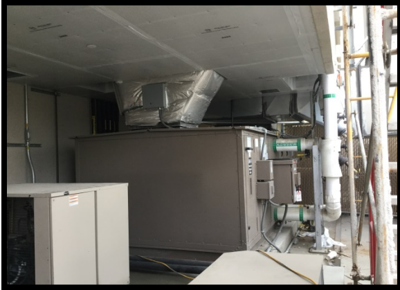
Level A IAHU #1 – Kitchen
