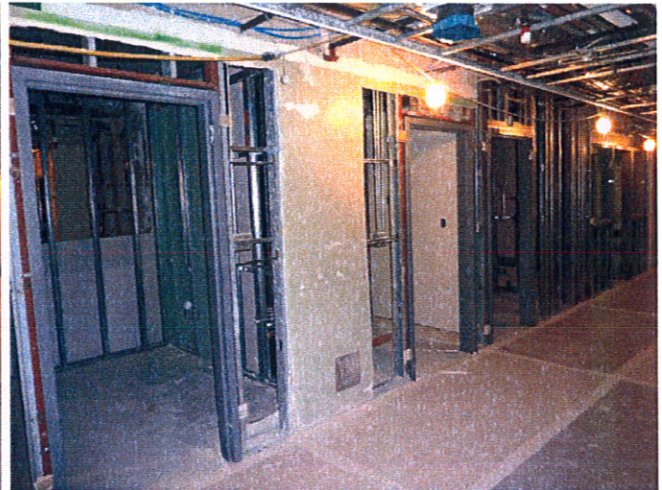
Photo #2: East Corridor
