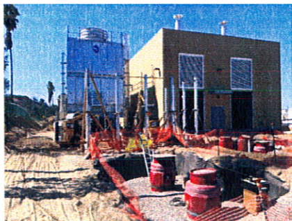
Fuel Tank and Screen Wall Posts
