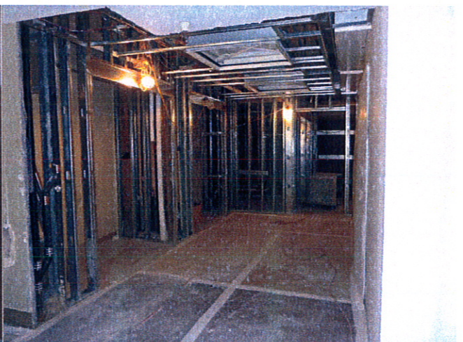
Photo #4: Elevator 5 & 6 Lobby
