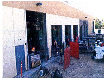
West Roll Up Doors & Piping Installation
