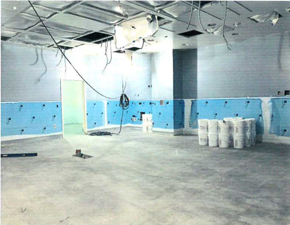
11-16-17: OR #1029 (Hybrid OR) Wall protection complete; installing finish flooring.
