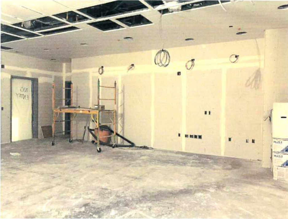
12-13-2017: Cath Lab 1024: ready for paint.
