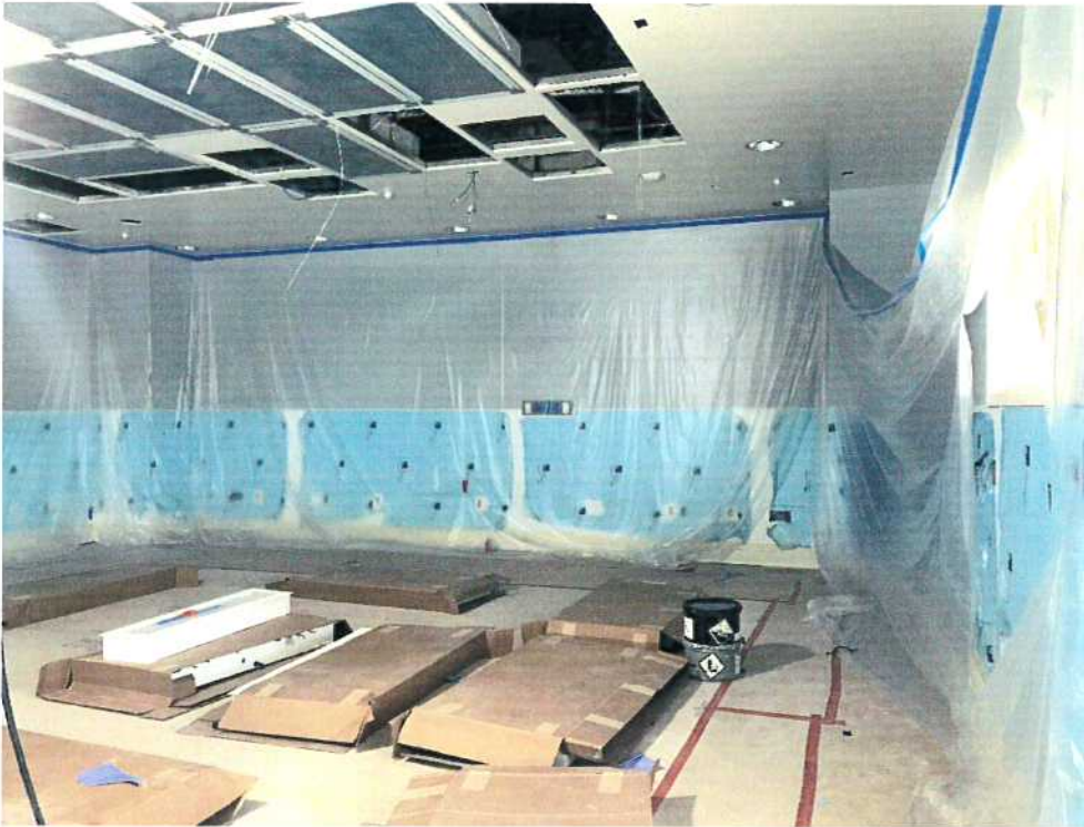
11-16-17: OR #1025 (General OR) Installing electrical fixtures and mechanical grilles.
