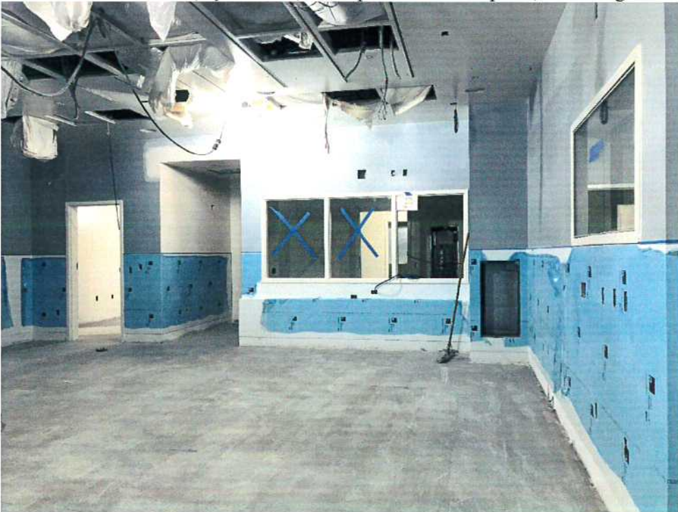
10-24-17: OR #1030 (Hybrid OR) Wall protection complete; installing finish flooring.
