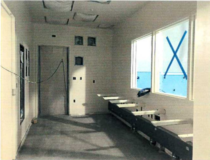
Control Room #1030A: Painted, installing finish flooring.
