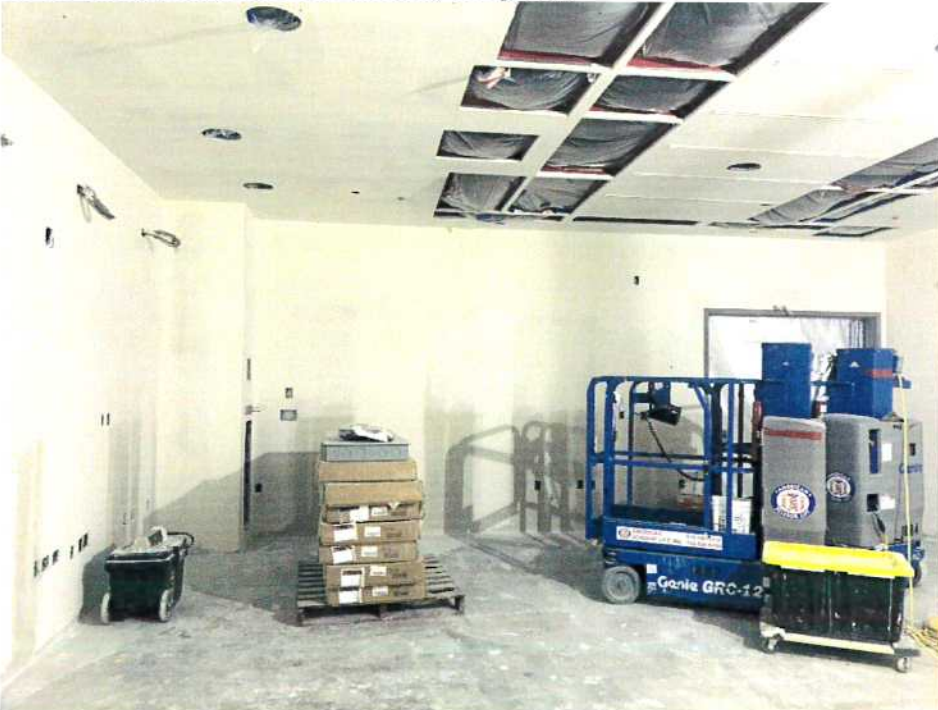
12-13-17: Cath Lab 1032: Prime coat painted.
