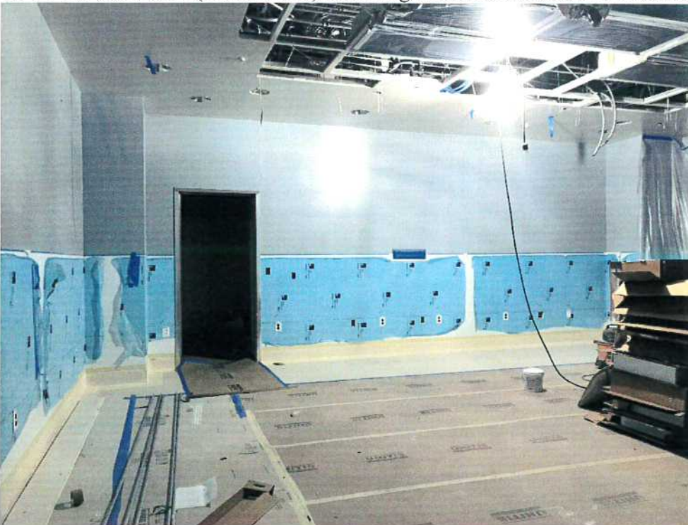
11-13-17: OR #1027 (Open Heart OR) Installing electrical fixtures and mechanical grilles.
