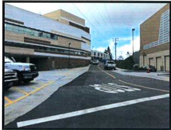
H&V Road Striping
