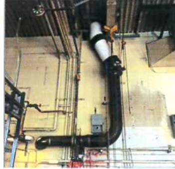
Final Chilled Water Tie-In
