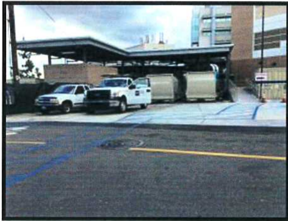
South Dock Concrete Backfill
