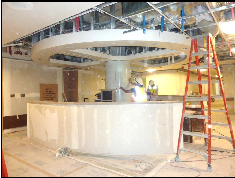
Central Nurse Station Progress
