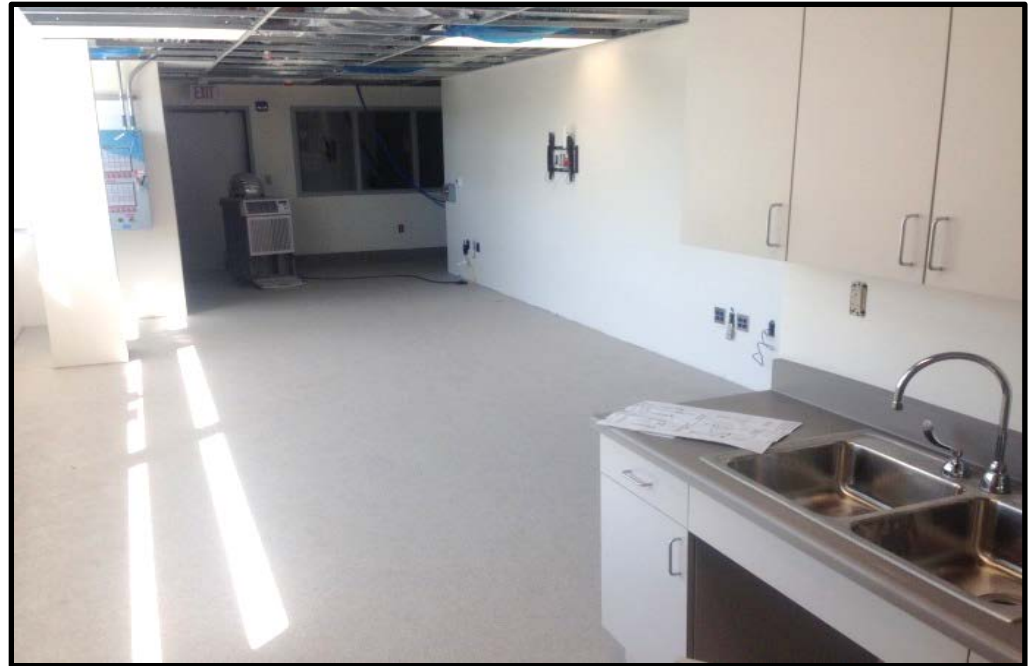
Control Room with flooring, casework, and countertop
