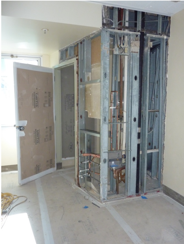
Photo #3: Patient Room Plumbing, ready for the new sinks
