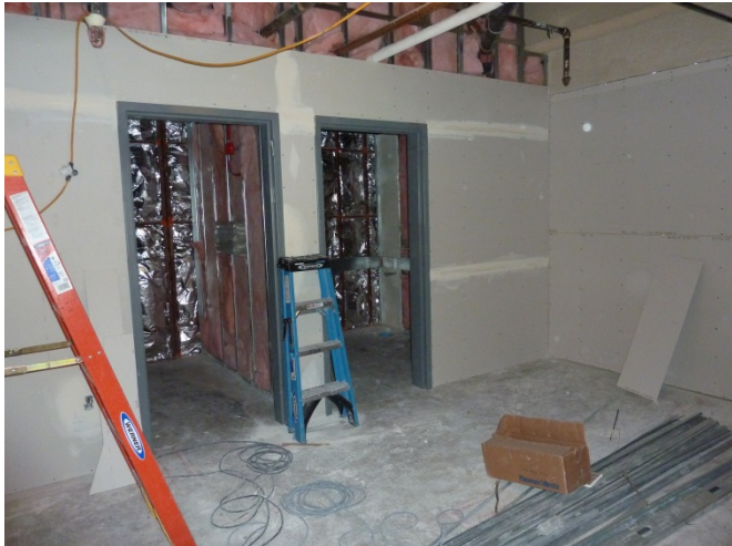
Photo #6: Staff Locker Room and Restrooms
