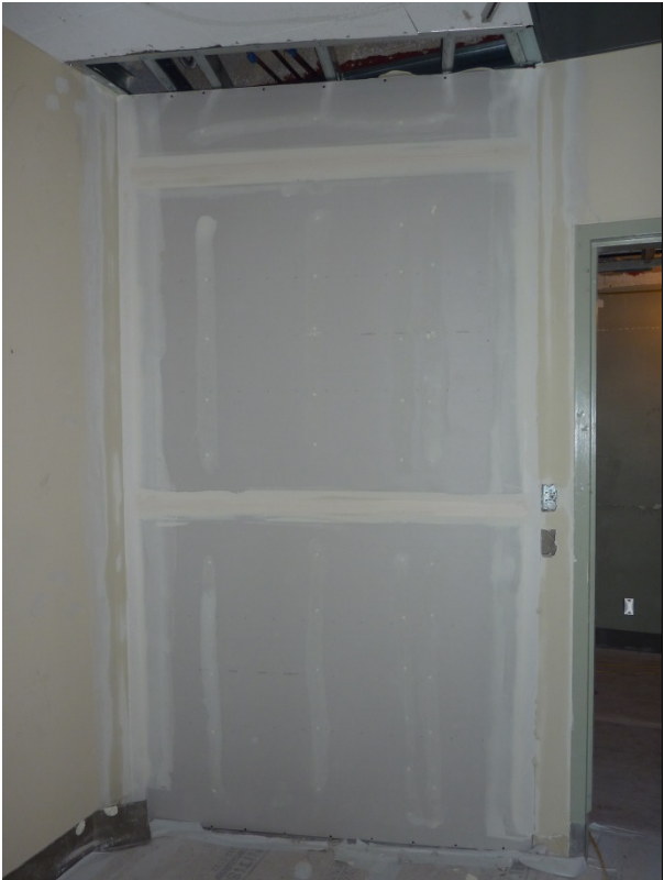
Photo #4: Patient Room Headwall prep
