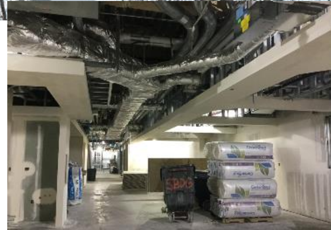
Overhead Utilities & Soffit Installation
