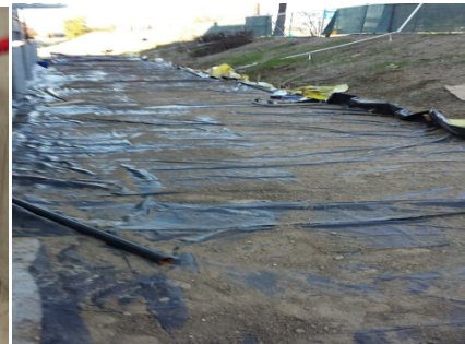
Pervious Concrete Curing
