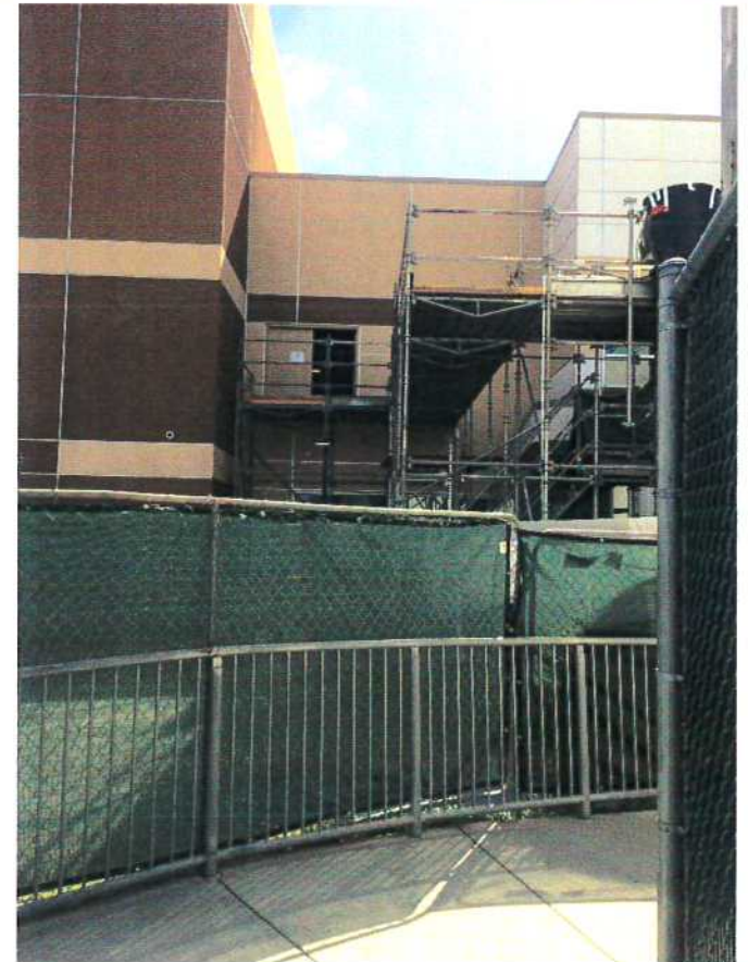
Scaffold Access to Level 1
