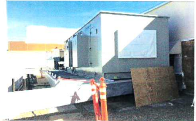
New Air Handler installation
