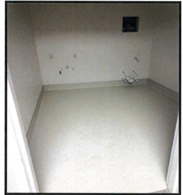
Level A Flooring Installation
