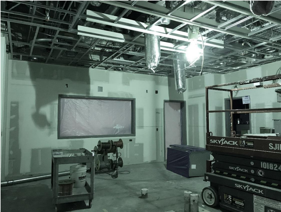
10-24-17: Cath Lab 1033: Drywall complete on walls.
