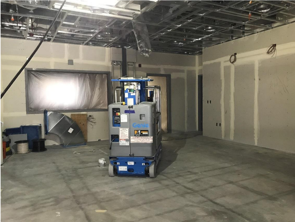
11-16-2017: Cath Lab 1024: ceiling framing complete.
