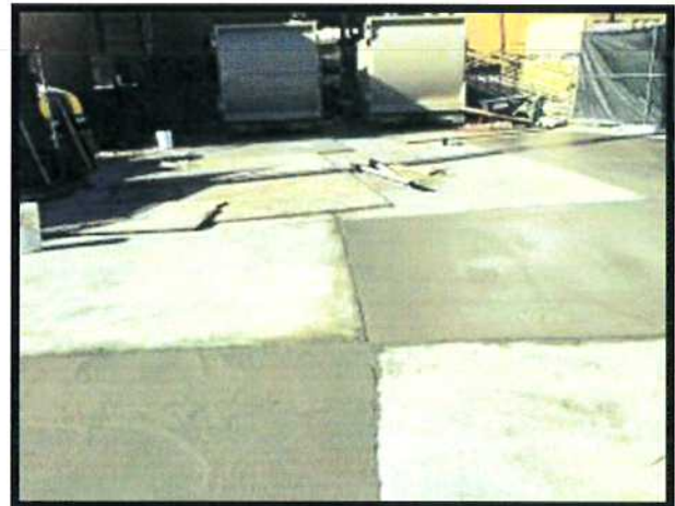
South Dock Concrete Backfill
