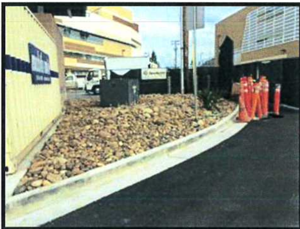
South Dock Landscape Cobblestone Install
