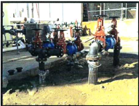
Helix Water Lateral Tie-In
