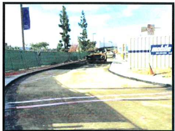
South Ring Road Asphalt Paving
