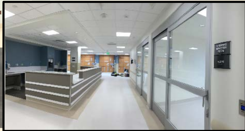
Central Nurse Control Station Casework Complete
