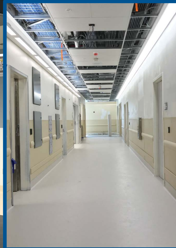
Southwest Corridor: T-Bar grid, wall protection, flooring, fire alarm devices installed
