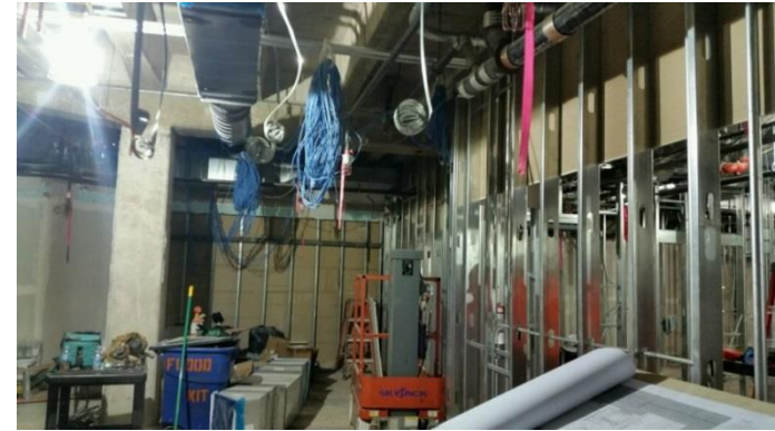
Drywall install for new Histology
