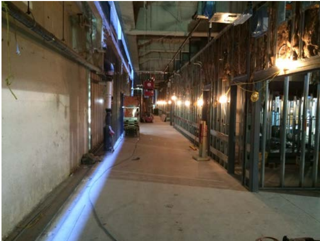
• Level B Framing MEP Systems
