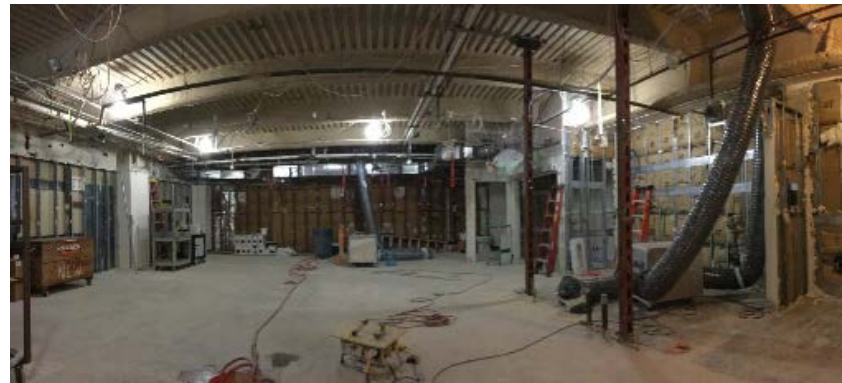
Demolition of Former Surgery Prep-B Space
