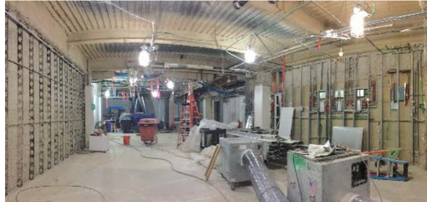
Demolition of Former Surgery Prep-A Space
