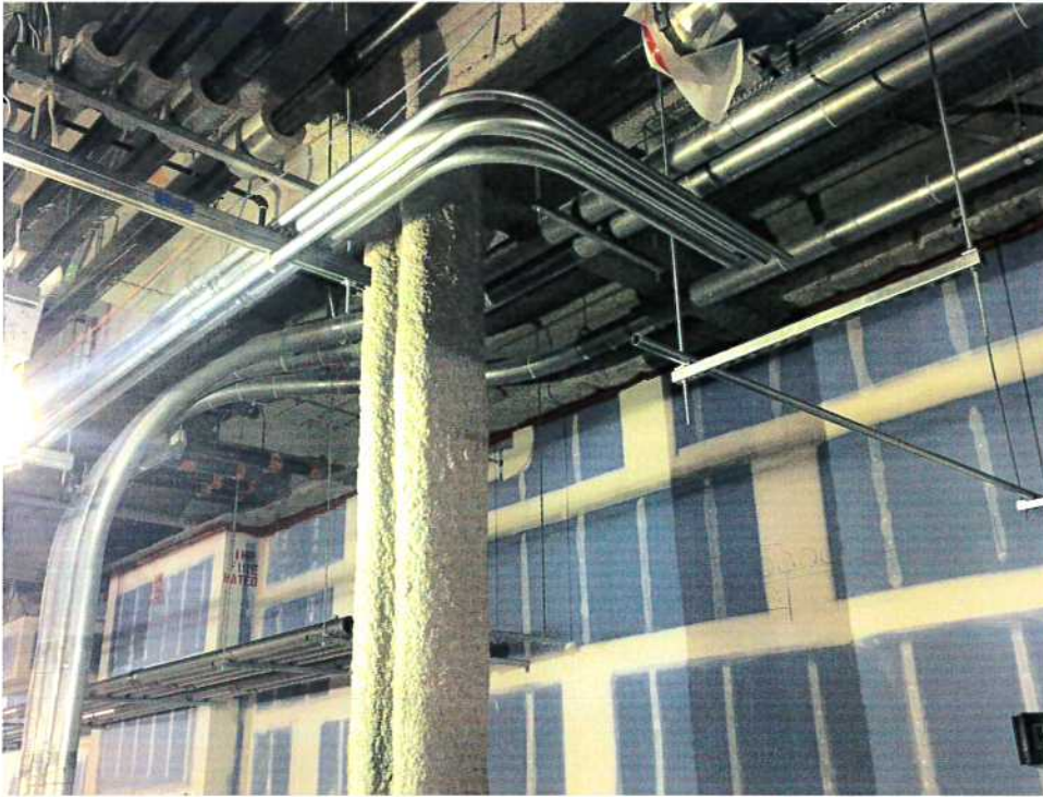
Electrical and low voltage conduits connecting to the Infill project
