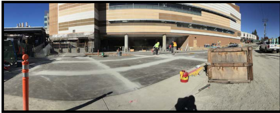
Loading Dock Concrete
