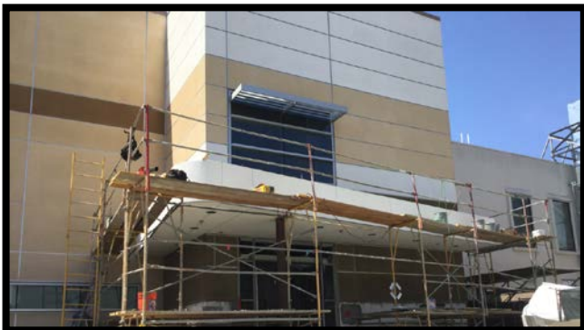
North Entrance Canopy
