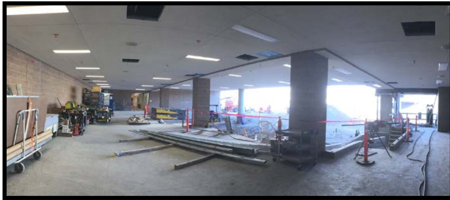
Loading Dock with Cement Plaster Ceiling
