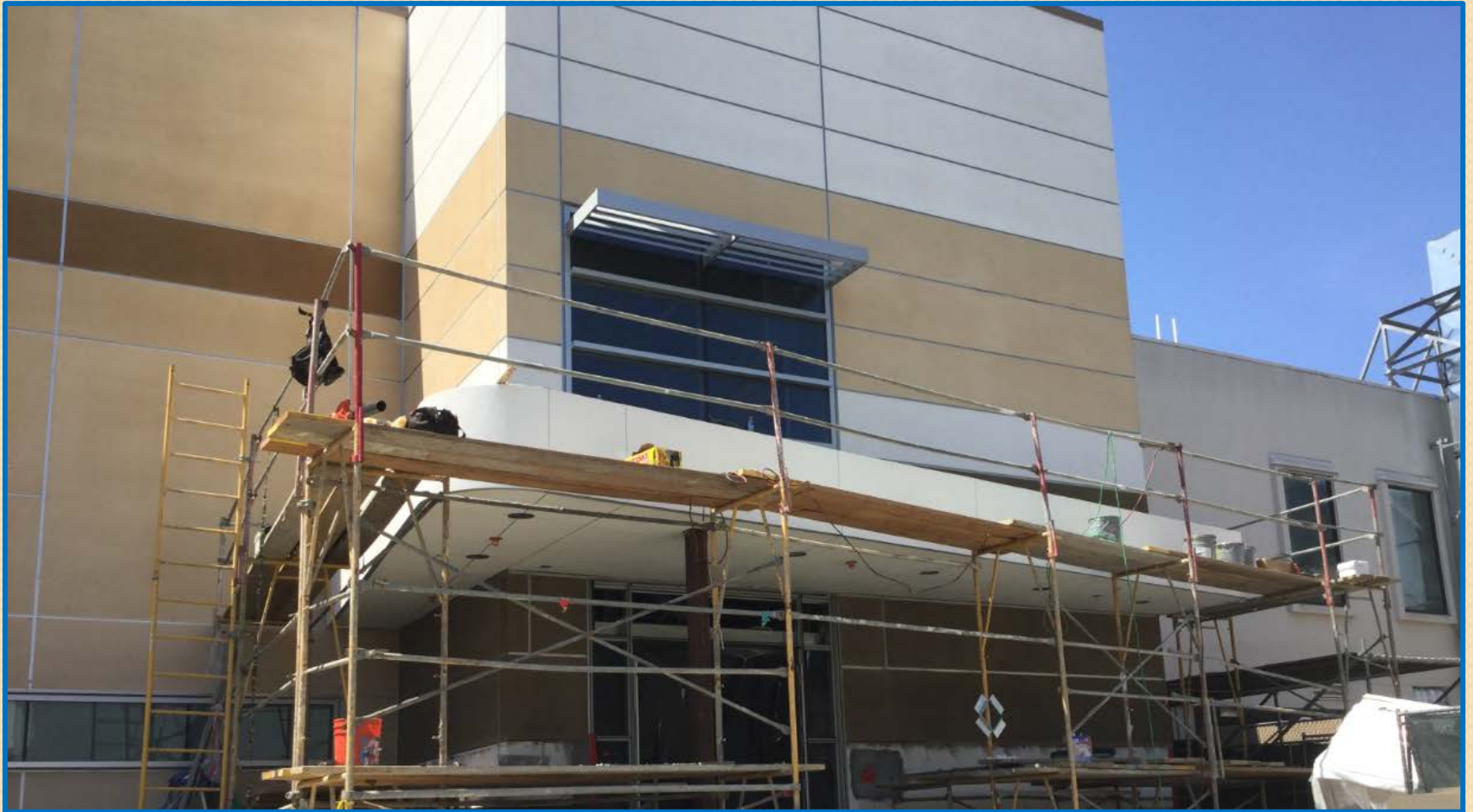
North Entrance Canopy
