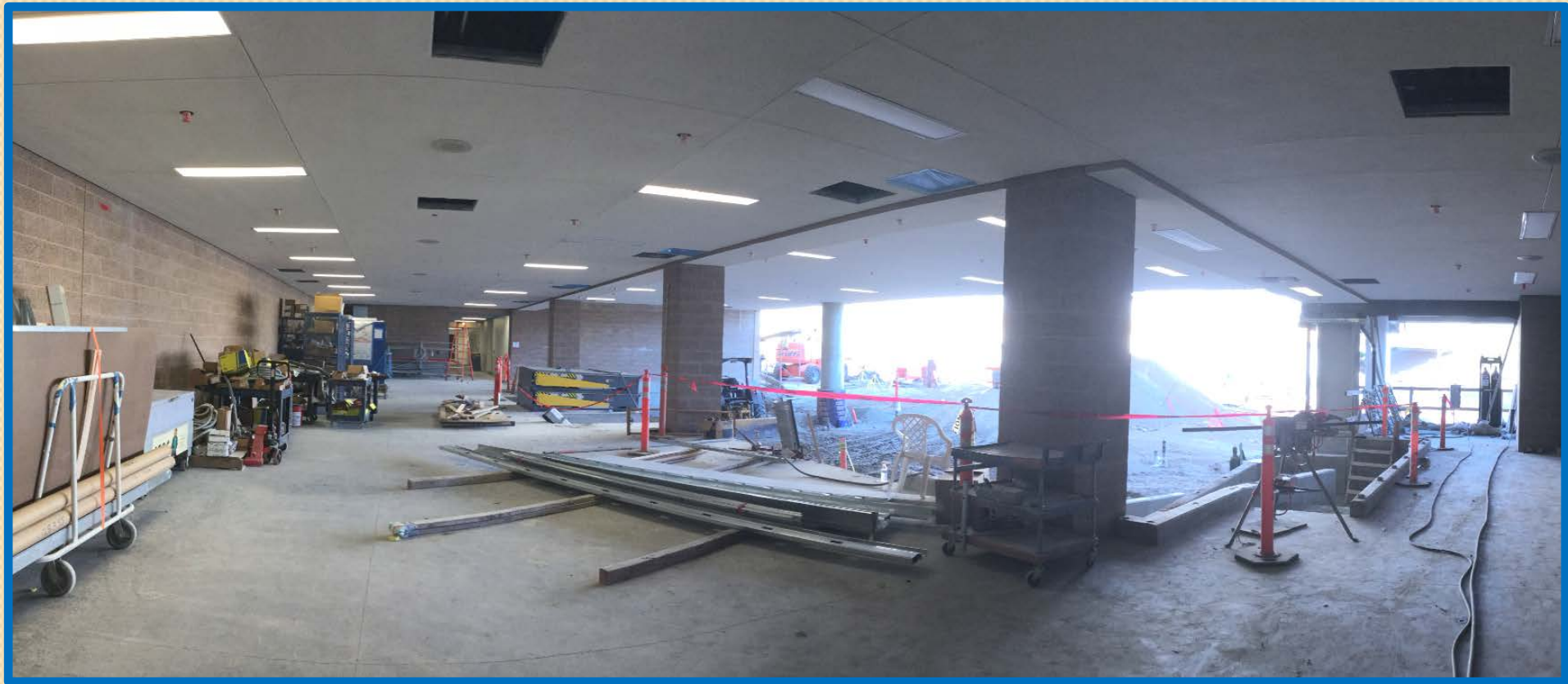
Loading Dock with Cement Plaster Ceiling
