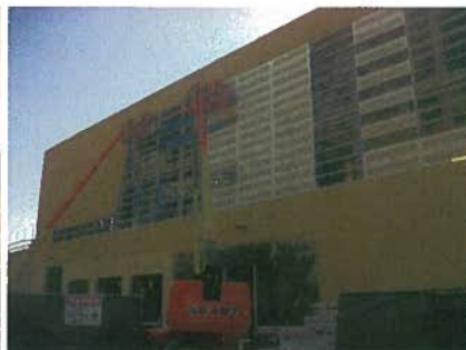
Curtain wall and Louver Installation
