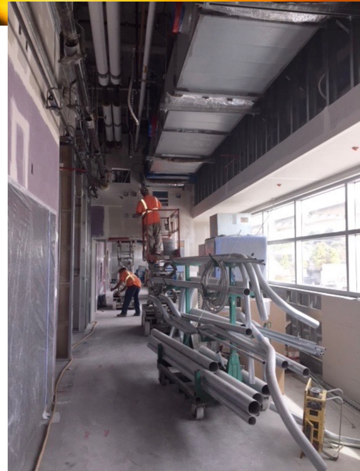
East Corridor: Overhead Utilities Installation is ongoing
