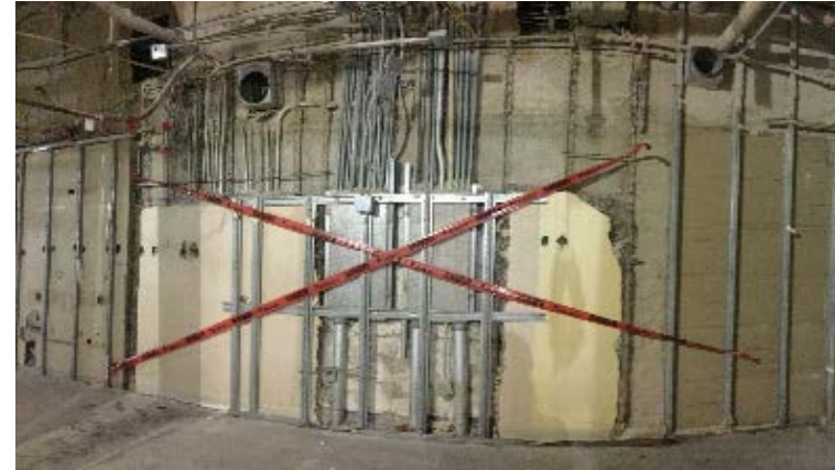
Level 1 Demo of Walls & Utilities
