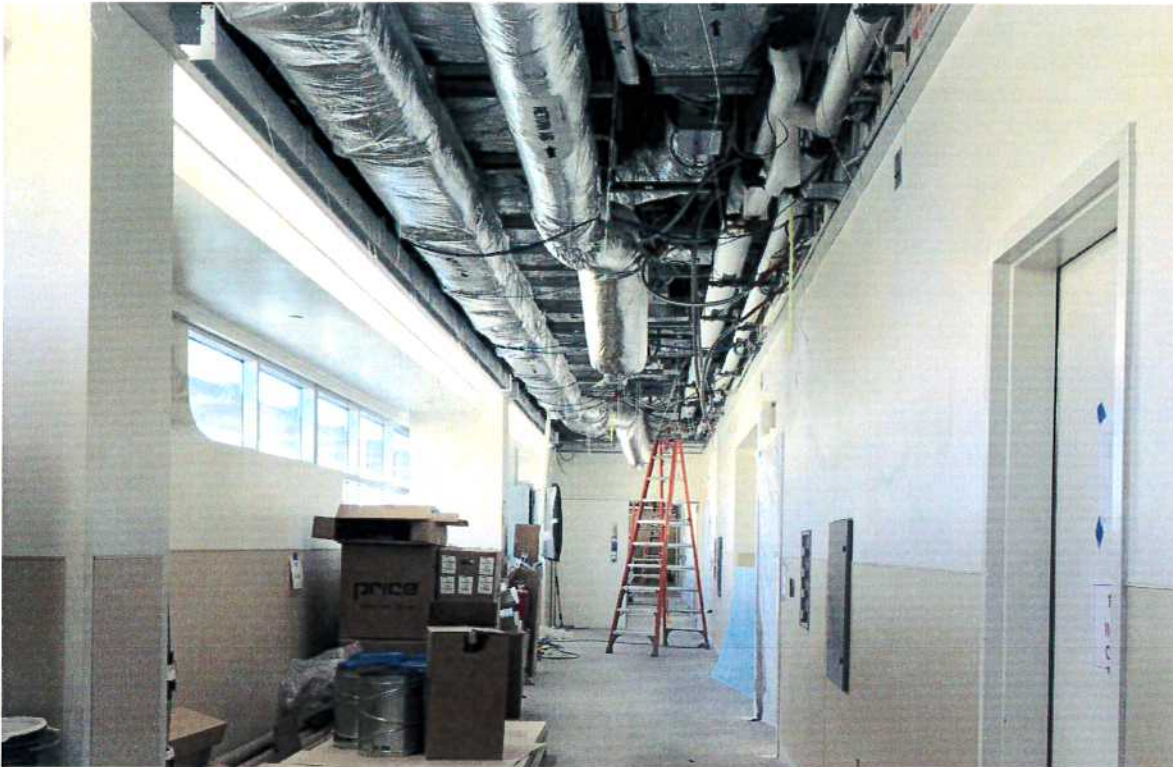
3-15-18: East Corridor: Wall protection installed. Getting ready to install T-Bar grid.
