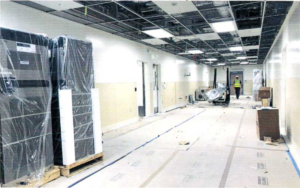
3-15-18: Sterile Core South: T-Bar grid/lights installed; medical equipment delivered.
