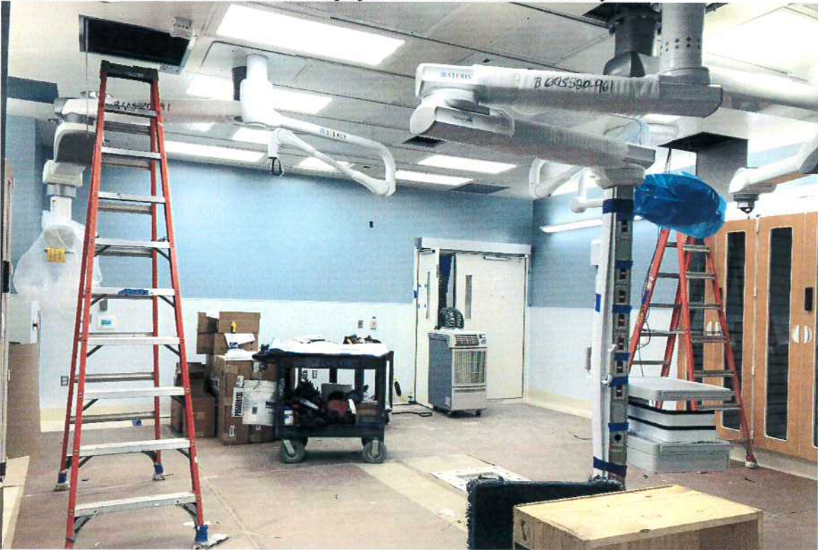
3-20-18: Cath Lab #1033: Medical equipment installation underway.
