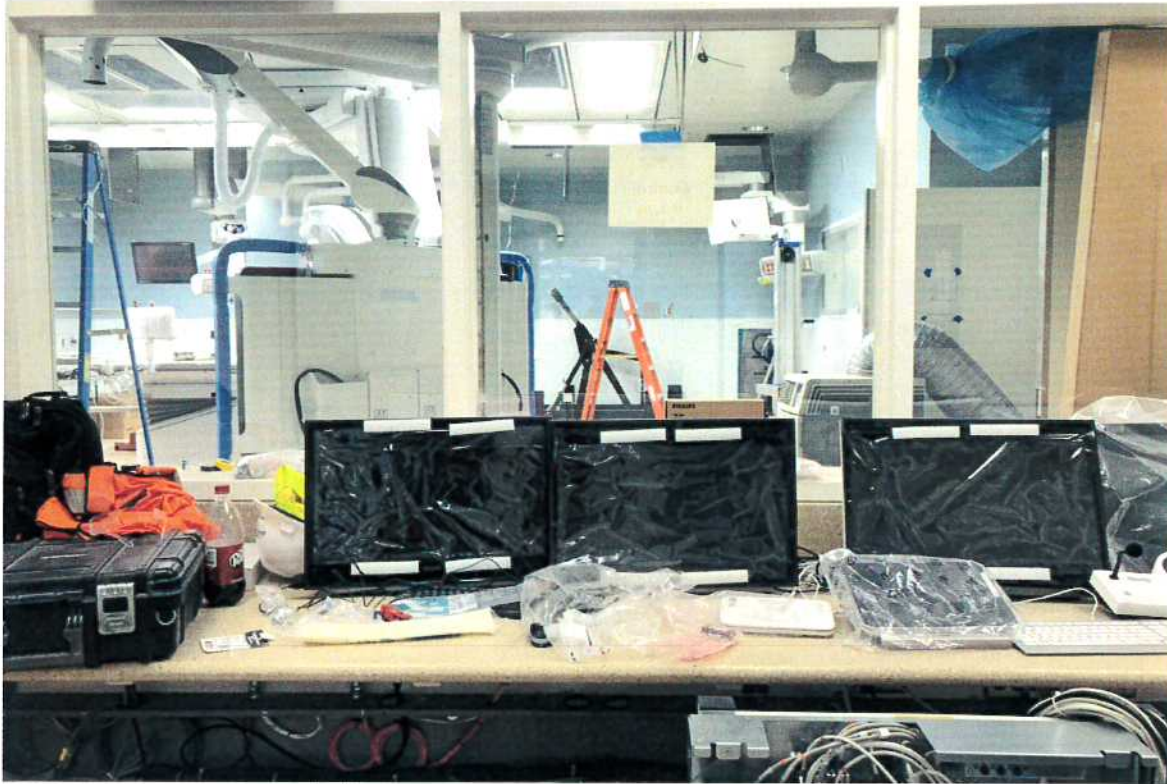
3-20-18: OR #1029 (Hybrid OR) Looking from the Control Room into the OR
