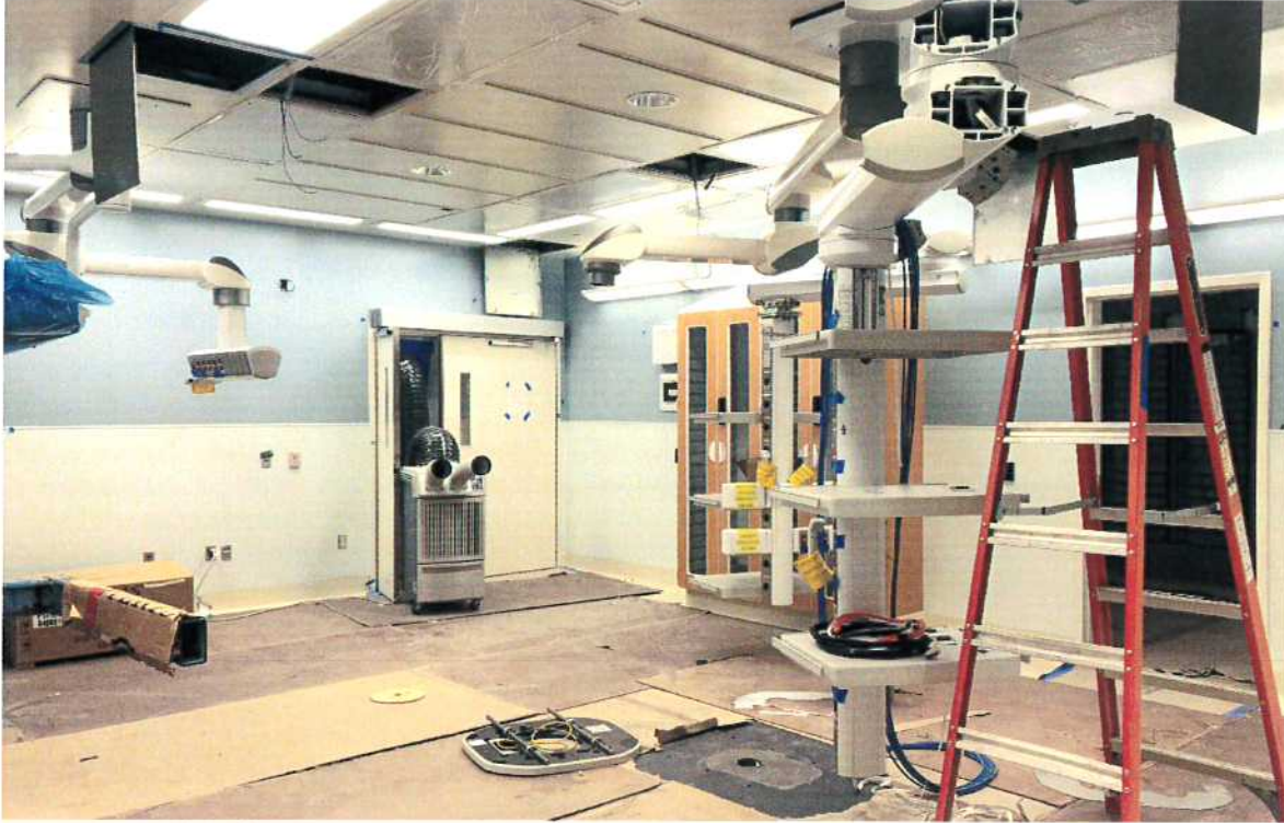
3-20-18: Cath Lab #1032: Medical equipment installation underway.
