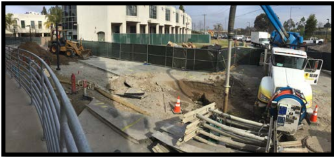
North Site Steam Line Work
