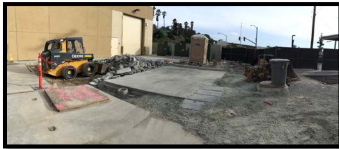
CEP and HV Site Coordination Work
