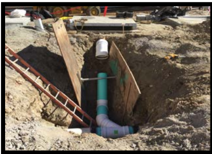
CEP and H&V Inlet Install
