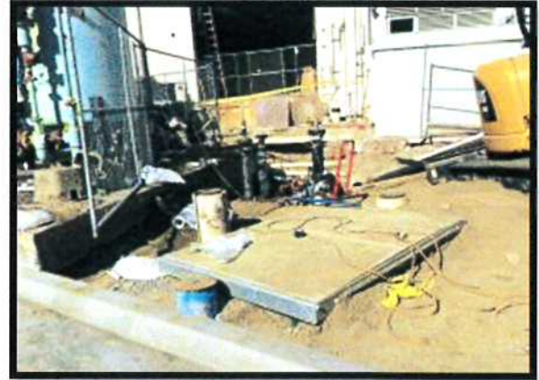
Helix Water Line Lateral Install
