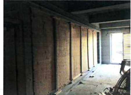
HVSB Wall with new column placed.
