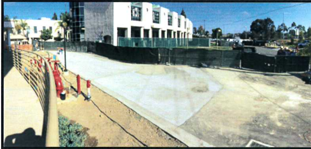
North Hardscape and Road Work
