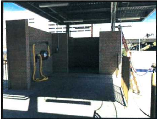
South Loading Dock Install
