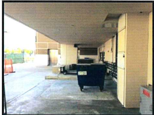
H&V North IAHU1 Ceiling Soffit Work
