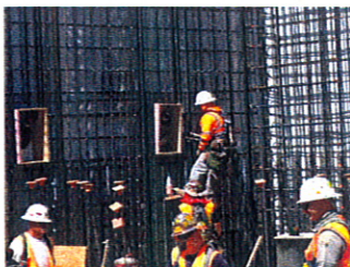
Reinforcing steel is set and ready for concrete in walls
