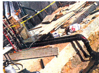
Under slab plumbing is installed
