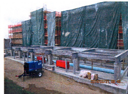
Cooling Tower Steel
