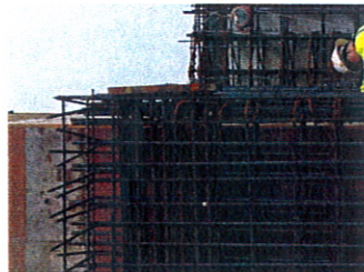
Reinforcing steel is set and ready for concrete in walls
