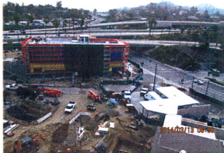
CEP & H&V from East Tower roof.
