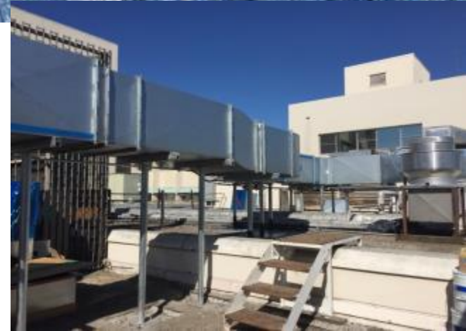
Air Handler & Duct Install
