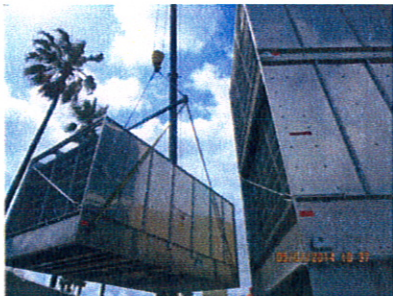
Cooling Tower Installation
