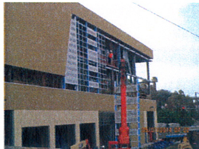
Curtain wall and Louver Installation
