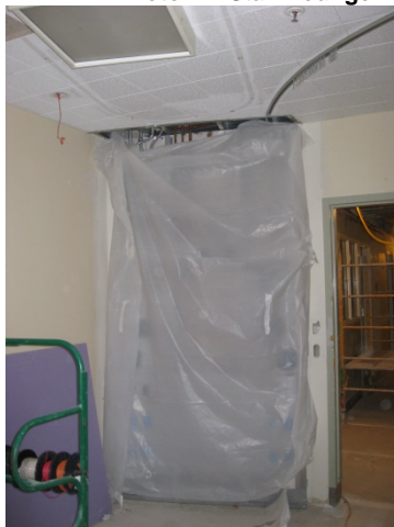
Photo #4: Patient Headwalls
