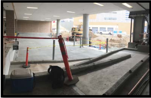
Loading Dock and Site Work
