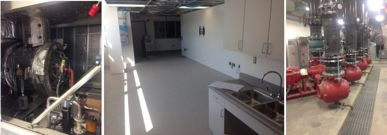
Solar On site to start Turbine Commissioning
