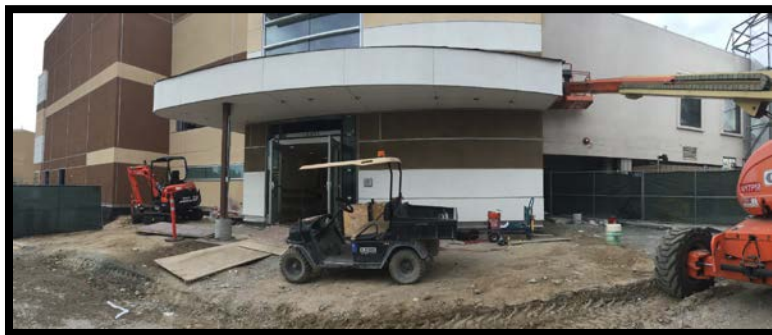
North Exiting and Site Work
