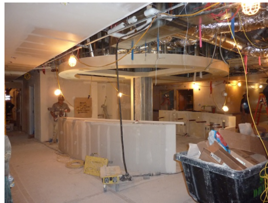
Central Nurse Station Progress
