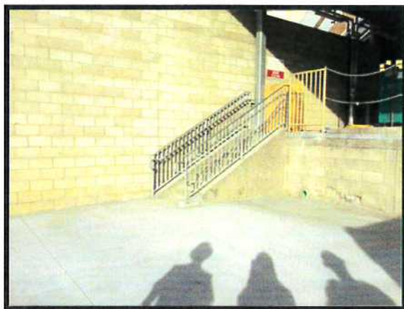
South Loading Dock Handrail
