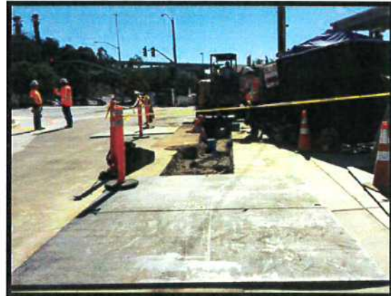
Helix Water Line Tie-in
