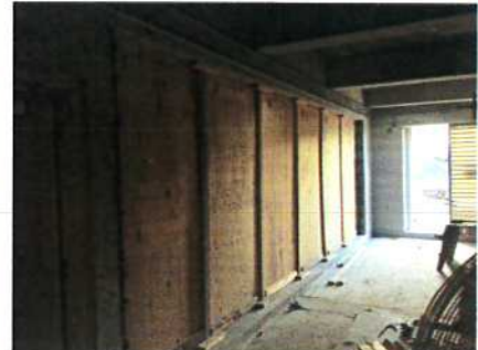
HVSB wall has been removed.
