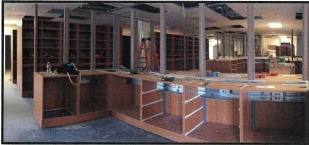
Pharmacy System Furniture Installation (RC Smith)
