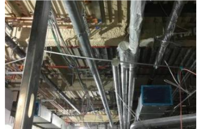
Overhead Utilities Installation
