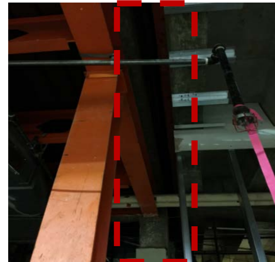
Existing overhead expansion joint
