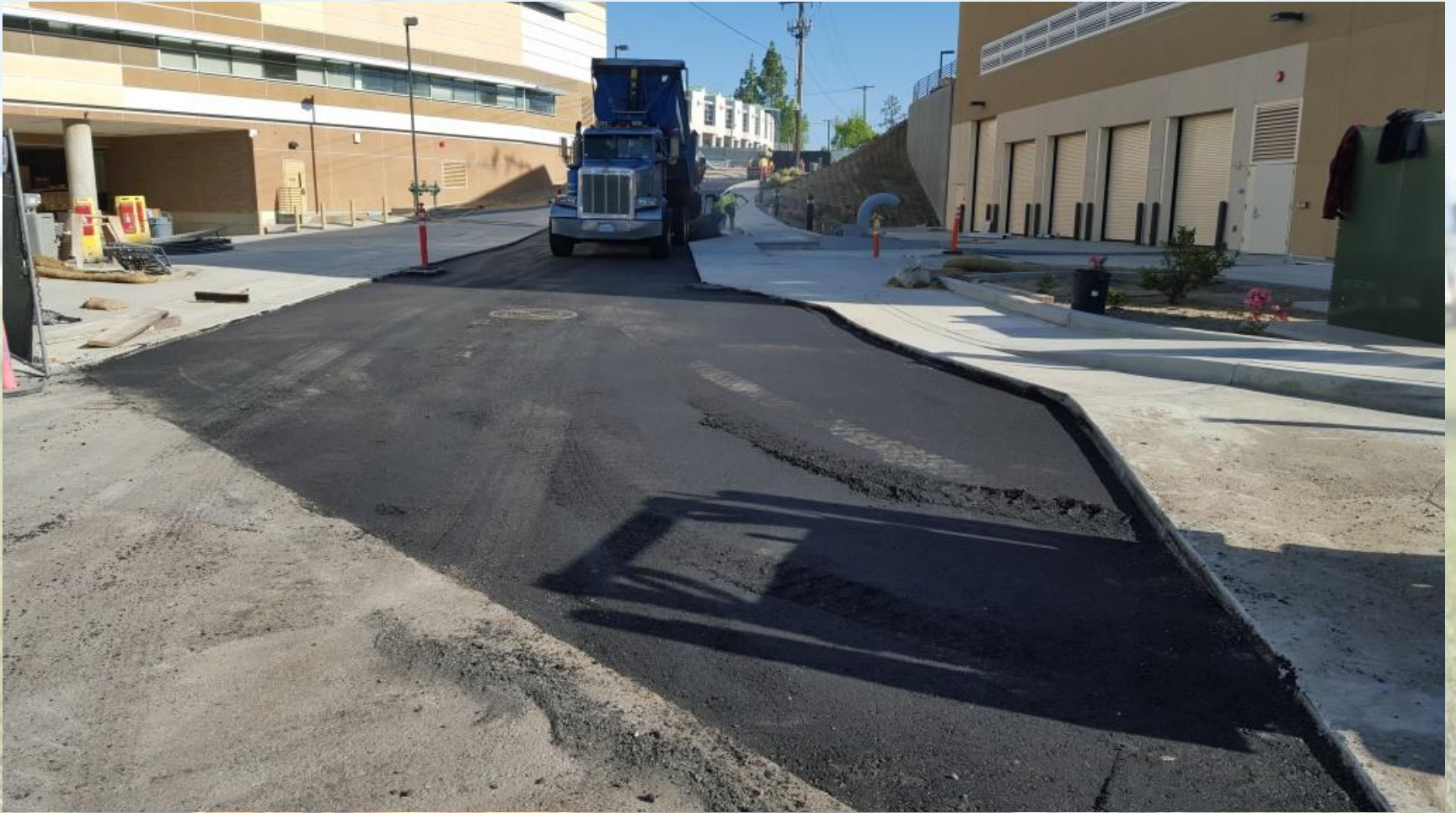
Asphalt Paving Between H&V and CEP
