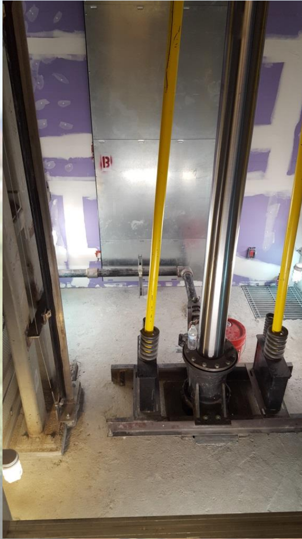
Elevator Pit Ready for State Inspection
