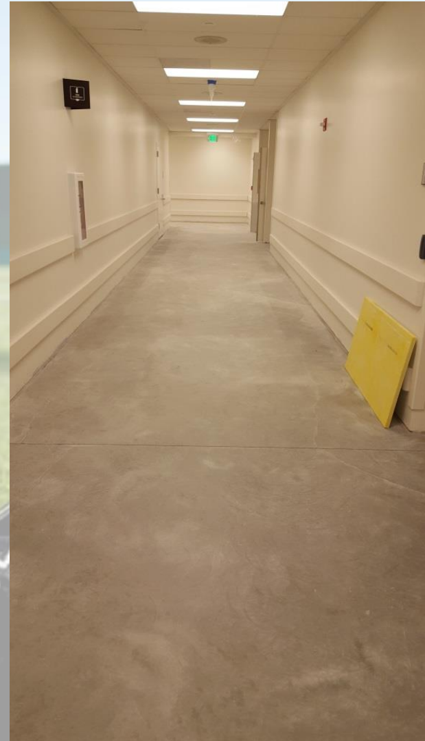
Level B Floor Ready For Clear Sealer
