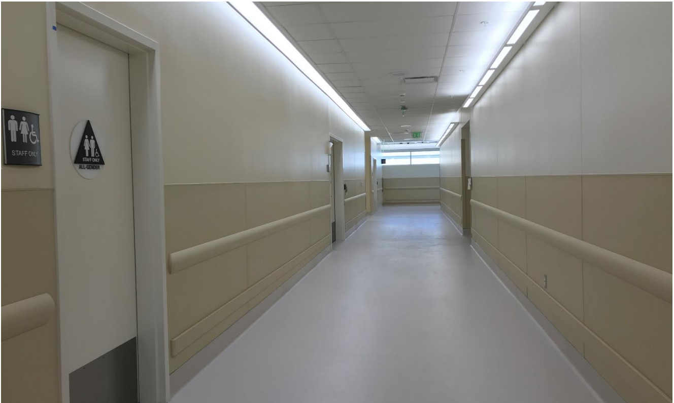
6-6-18: North Corridor complete.
