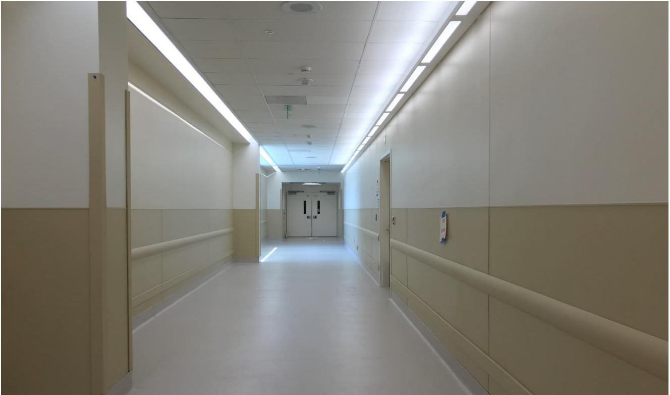
6-6-18: South Corridor complete.
