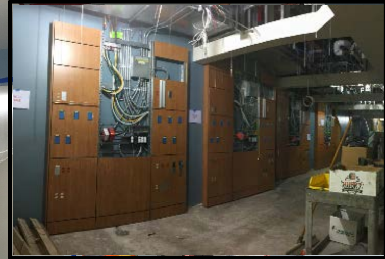
PACU 1 Headwall Installation
