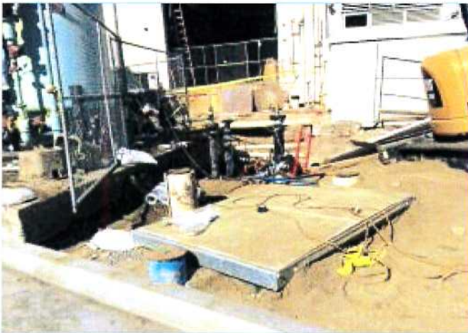
Helix Water Line Work
