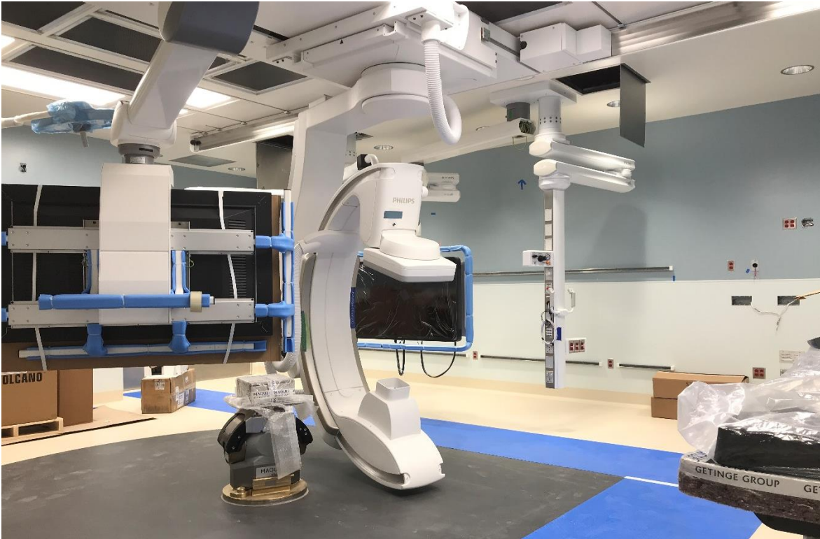
4-24-18: OR #1030 (Hybrid OR) Wrapping up the medical equipment installation.
