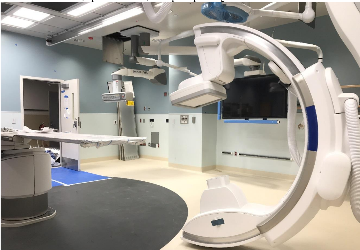
4-24-18: OR #1029 (Hybrid OR) Medical equipment installation nearing completion.
