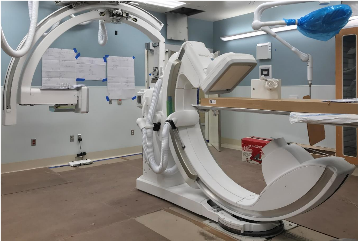
4-24-18: Cath Lab #1033: Medical equipment installation nearing completion.
