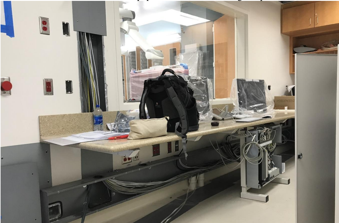
4-24-18: Cath Lab #1033A Control Room.
