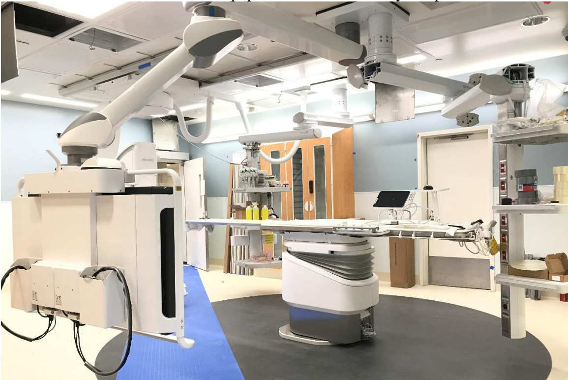
3-20-18: Cath Lab #1032: Medical equipment installation nearing completion.
