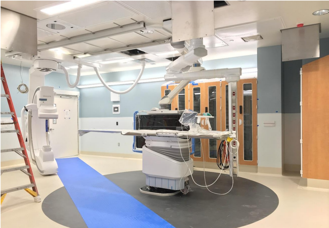
4-24-18: Cath Lab #1024 Medical equipment installation nearly complete.
