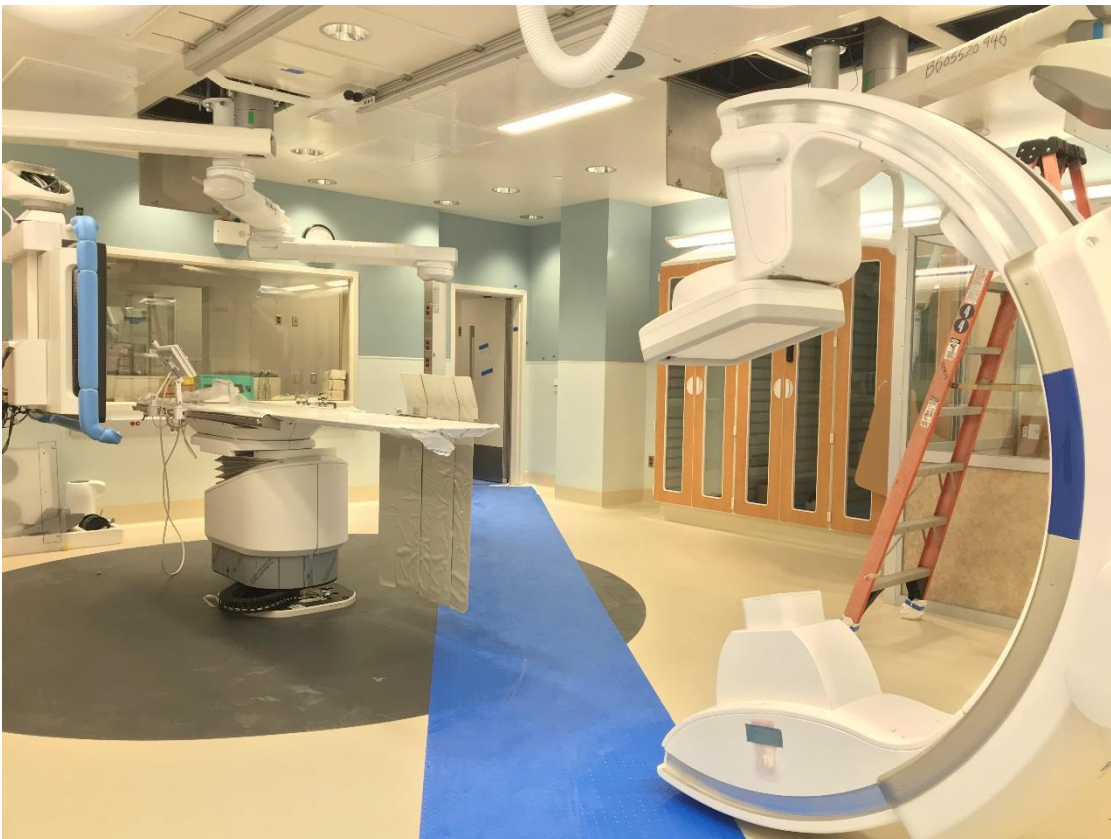
4-24-18: Cath Lab #1023 Medical equipment installation nearly complete.
