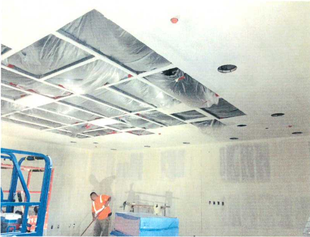
10-24-17: OR #1025 (General OR) Drywall ceiling installation complete, ready for paint.
