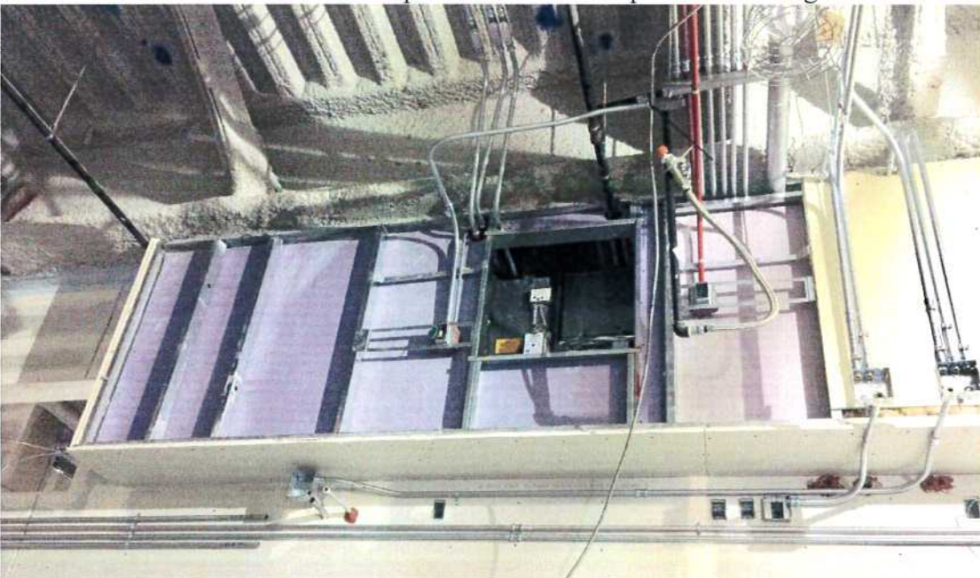
10-24-17: Relocated Smoke Fire Damper access complete for existing AHU-22
