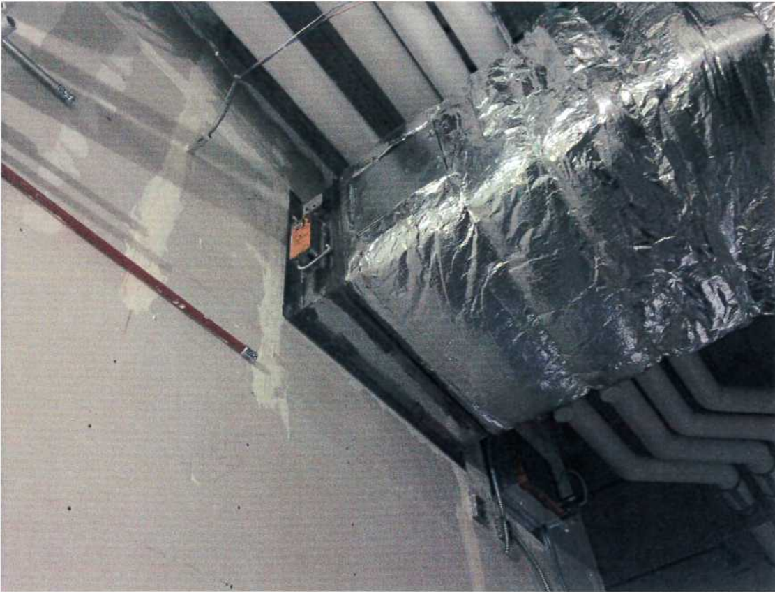
10-24-2017: New Smoke Fire Damper Installation complete on existing AHU-22
