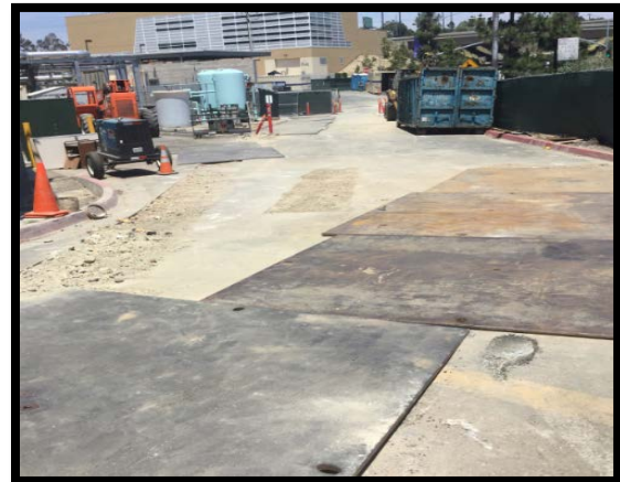
Helix Water Line Pot Holing
