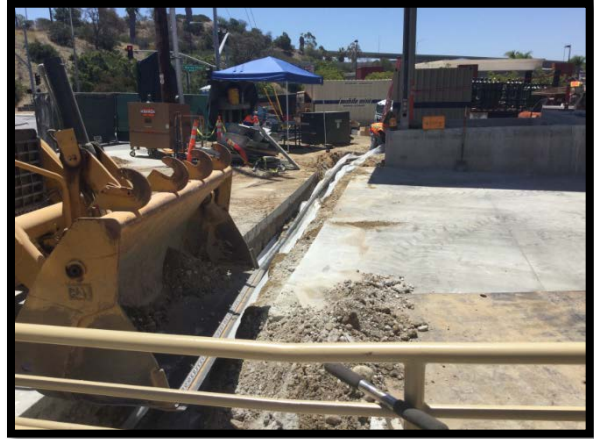
South Loading Dock Sewer Install
