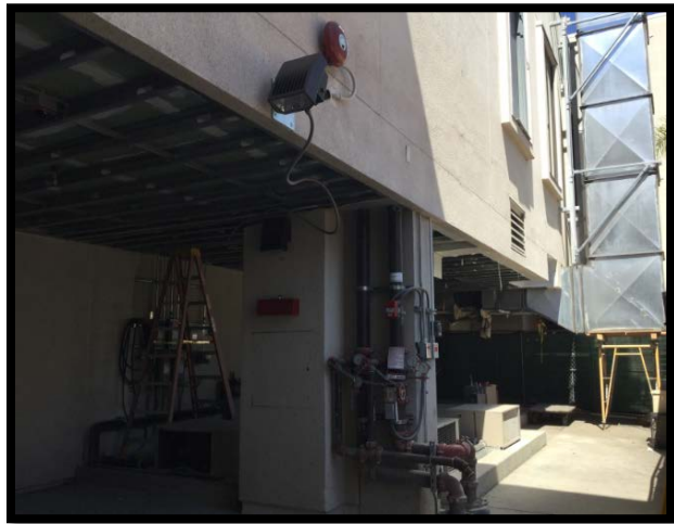
H&V North IAHU1 demo and Ceiling Work
