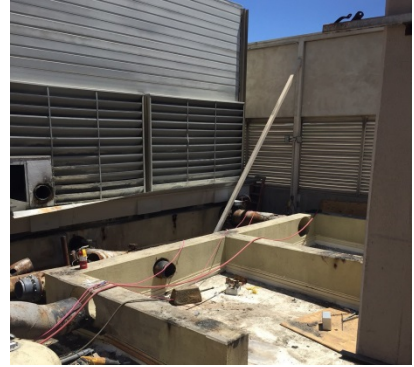
Demolition existing cooling towers
