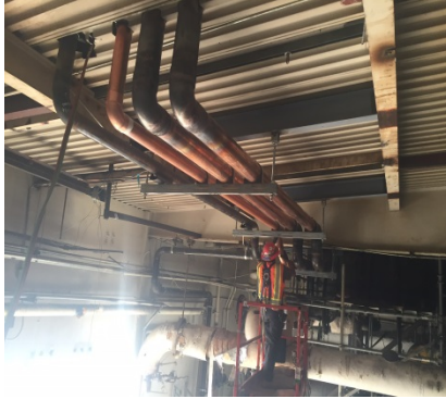
Medical gas and soft water lines being installed
