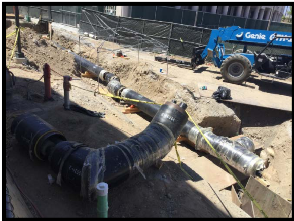
North UG Steam Line Install
