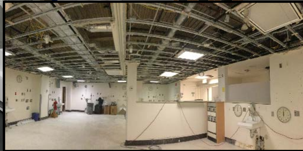
Start Demolition of former Prep B
