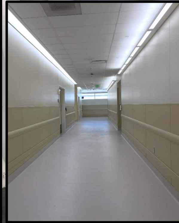
North Corridor: Complete
