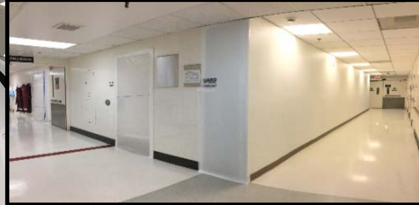
Phase 3 Barrier Install
