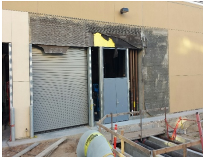
Wall enclosure above utility tunnel
