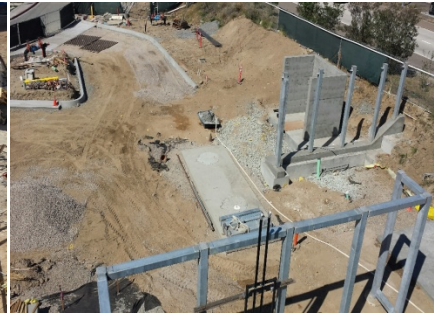
North site curb & gutter and trash enclosure
