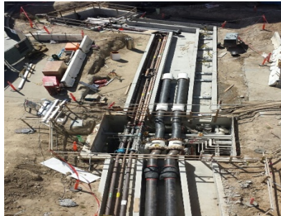
Utility Tunnel being fitted out with piping
