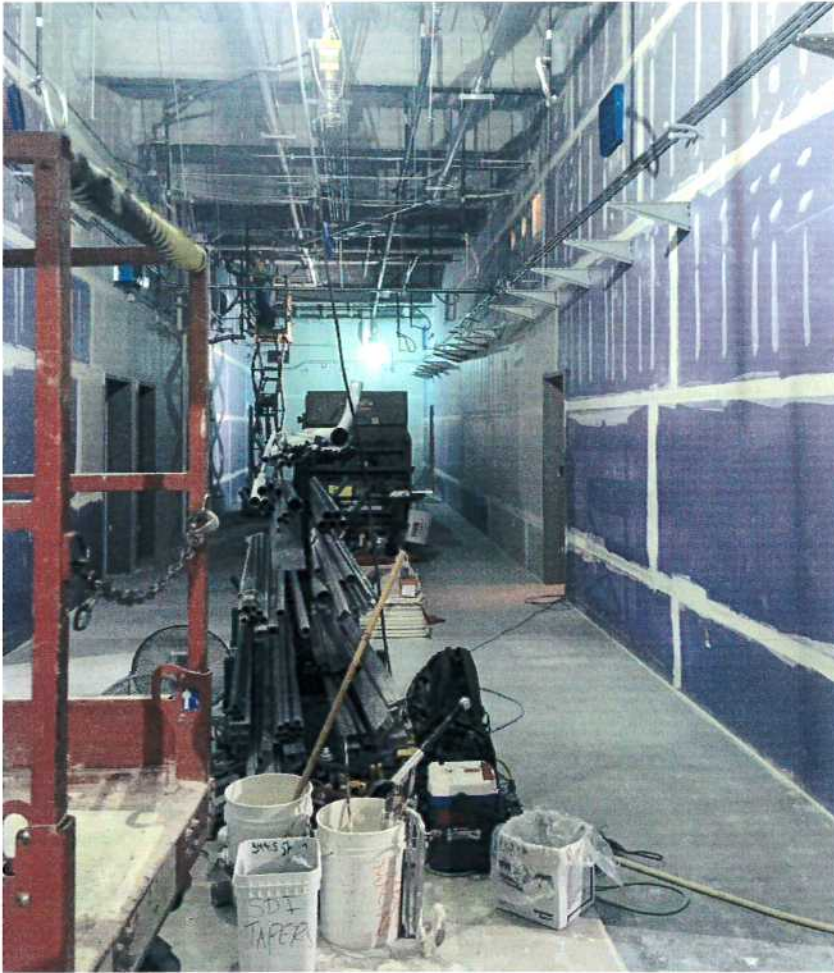
8-17-17: Ongoing work at Central core
