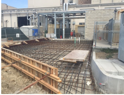
Rebar at new O2 Farm
