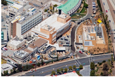
New Aerial Photo of the new H&V and CEP
