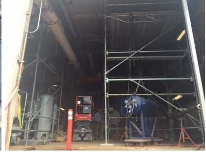
Demolition of Equipment in Existing Plant
