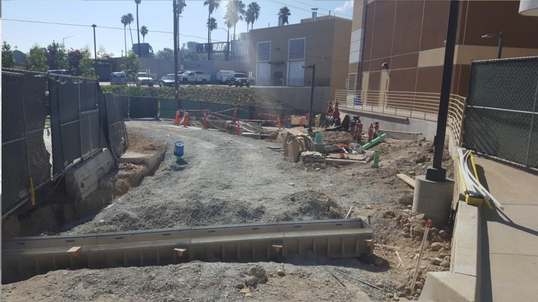
North Steam Line and Hardscape Preparations
