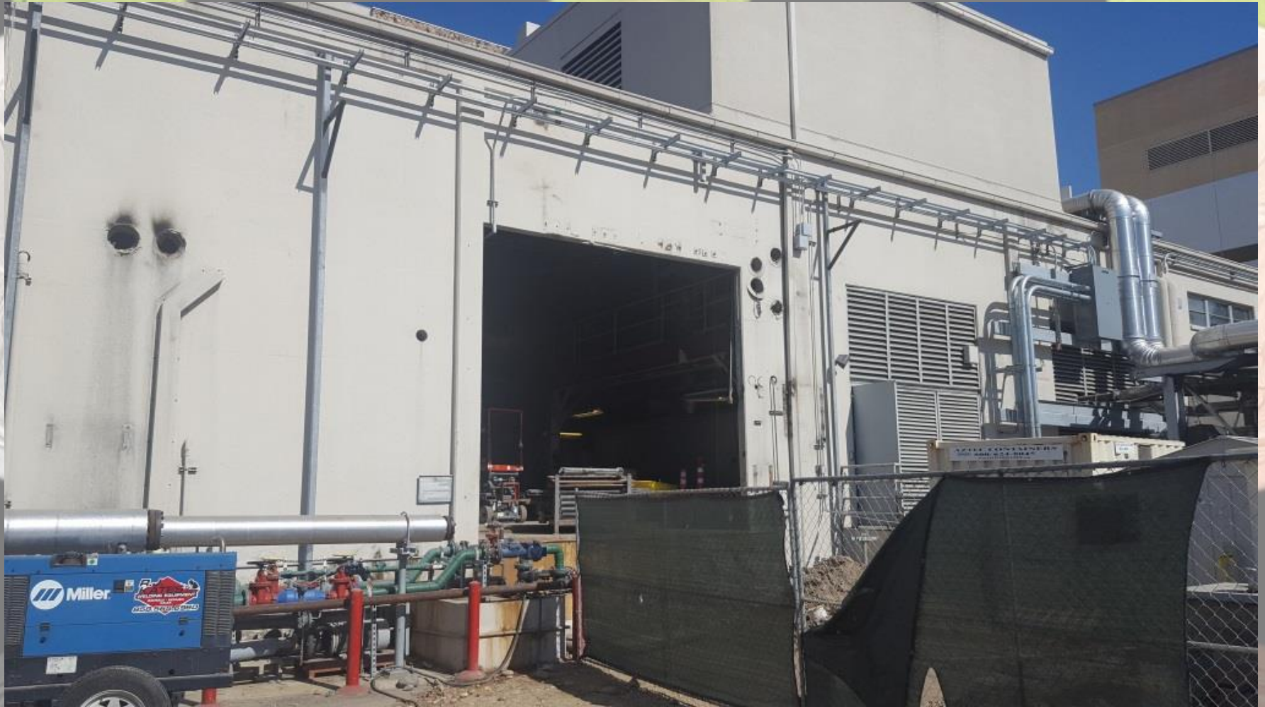
Demo of Existing Systems
