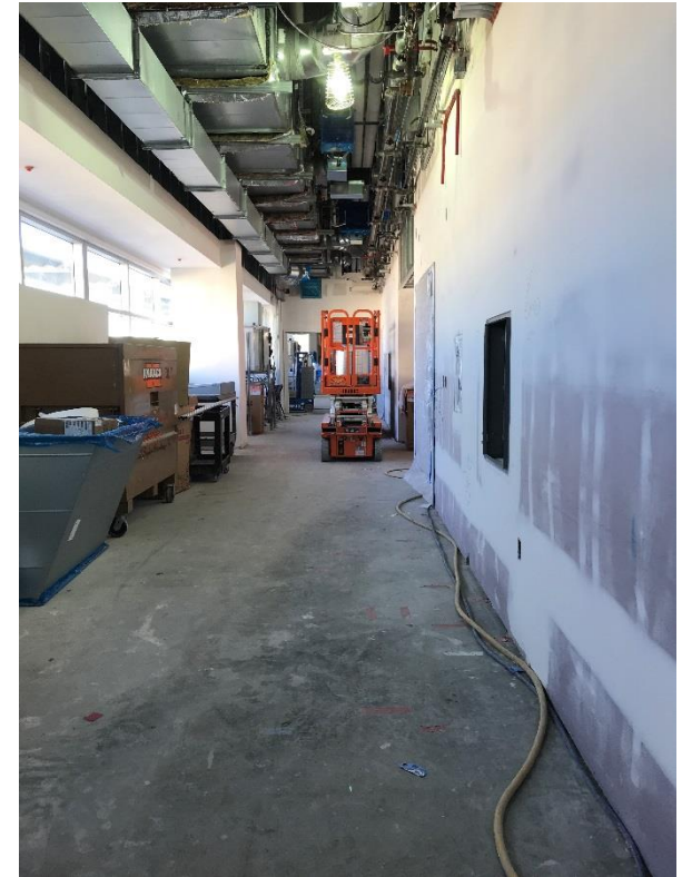
East Corridor: Overhead Utilities nearing completion; drywall complete; painting underway
