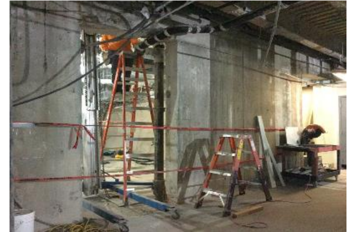
Level 1 Shear Wall Demo
