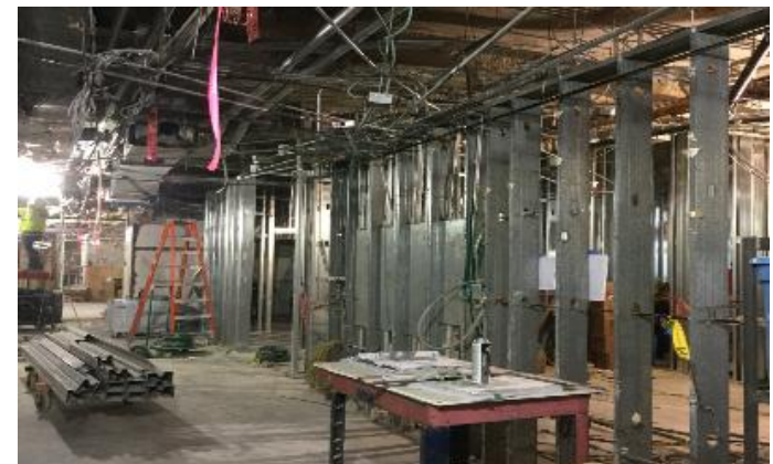
PACU 1 Wall Frame Installation
