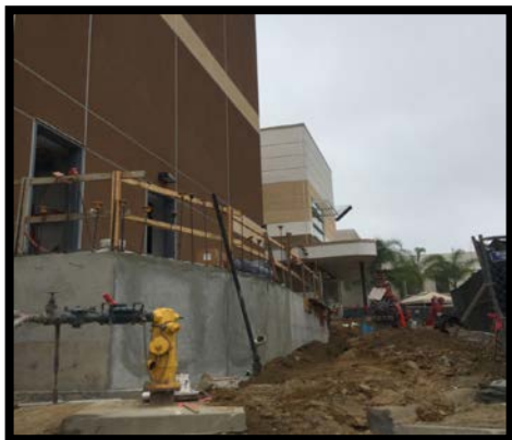
North Exiting Ramp
