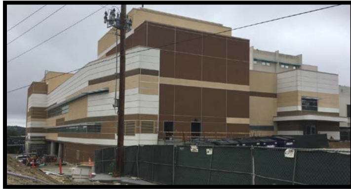
Exterior Building Skin Refinish
