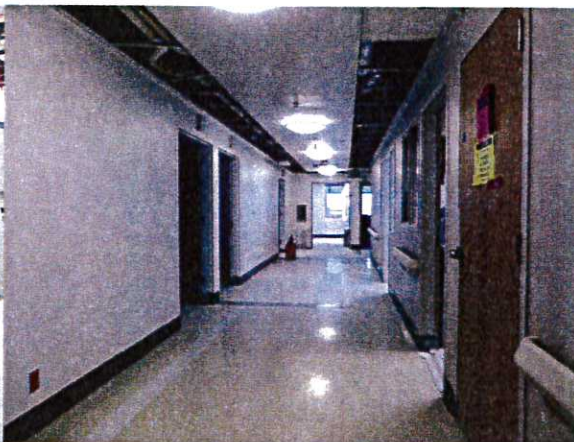
Photo #2: Corridor ceilings
