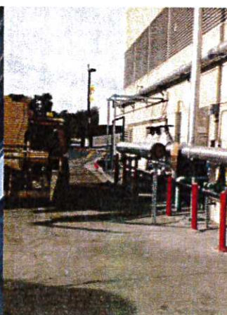
Temp Boiler being removed
