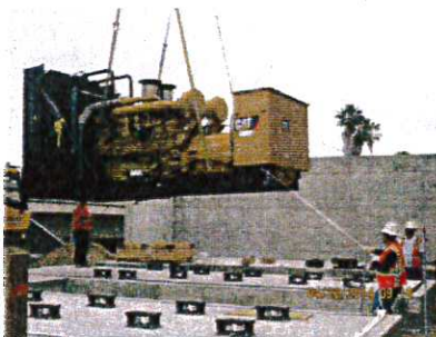
Emergency Generator Installation
